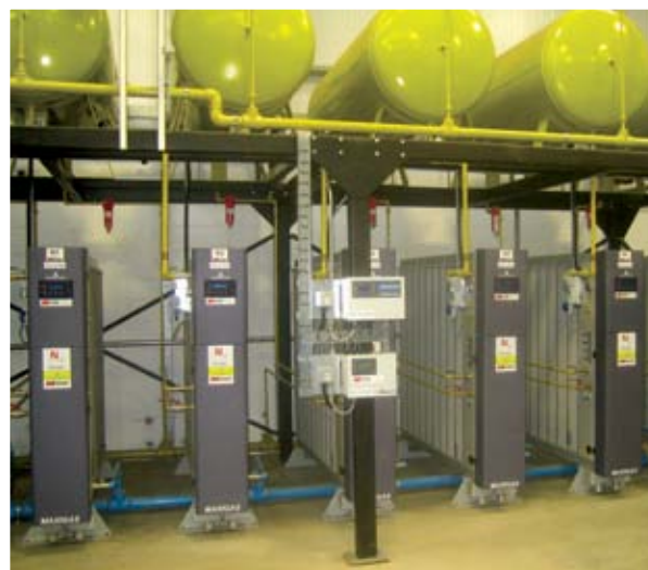
A six bank MAXIGAS installation. (Five generators in view) satisfy the peak demand, each capable of supplying 20% of the output. The banks cascade on and off load as the flow varies with factory production requirements. This saves significant energy costs during low flow periods, in the form of lower compressed air demand. The sixth bank provides 100% back-up and allows for 100% up-time during maintenance.
